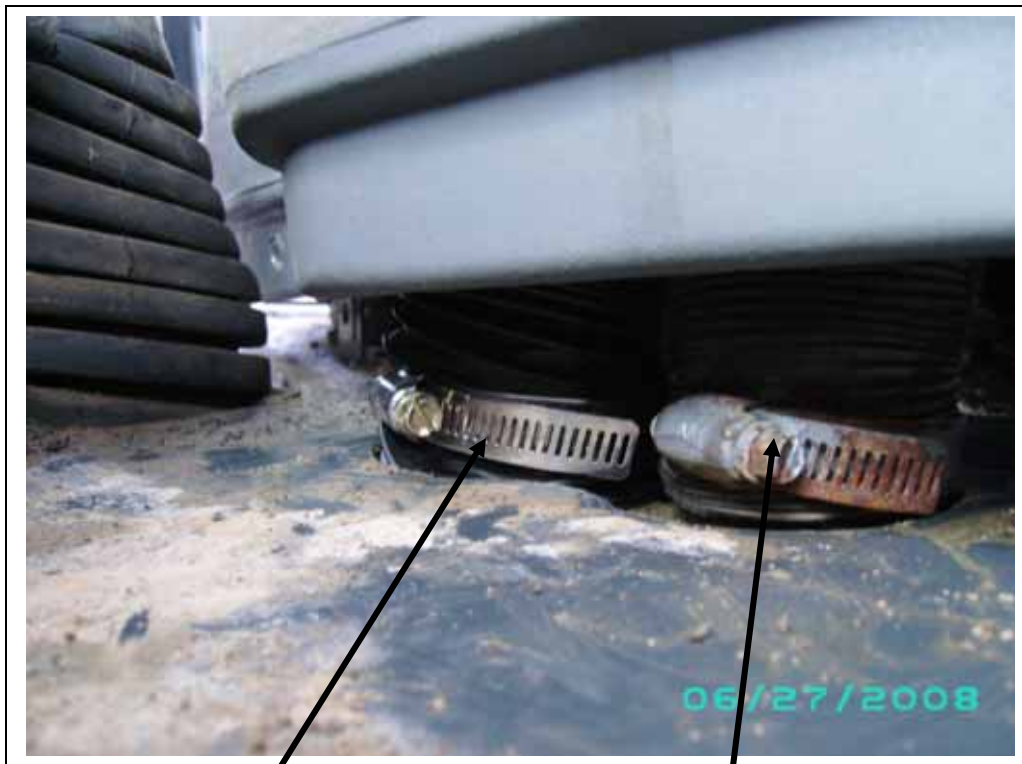
New 2 ½" flex duct installed using a #40 gear clamp.
