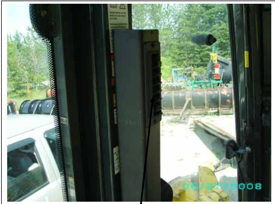
Rectangular louver installed once the square duct is secured.
