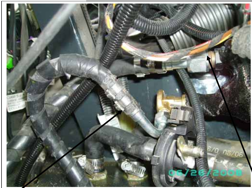
Heater lines reconnected with evap box in place.
